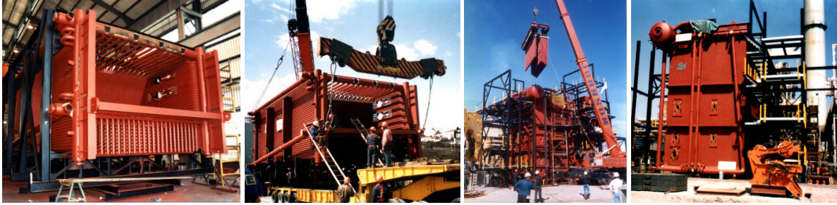
FIGURE 4. Manufacturing, transport, and installation of a 120 t/h, 400°C and 42 bar gas and oil fired water tube boiler in Cape Town, South Africa.
