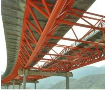
(b) The bridge truss
