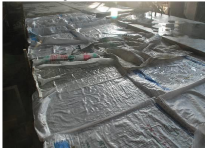
(c) Pouring concrete deck
