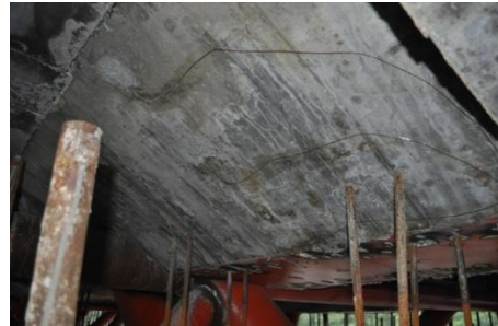
(b) Measurement points on the concrete deck
