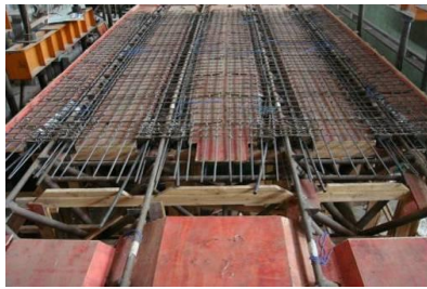
(b) Lashing and embedded steel bars
