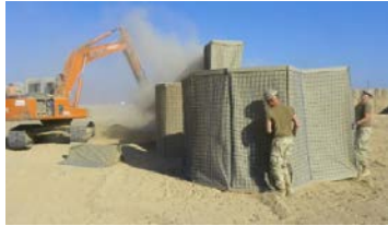
Fig. 3: Building Delaram FOB [87]
