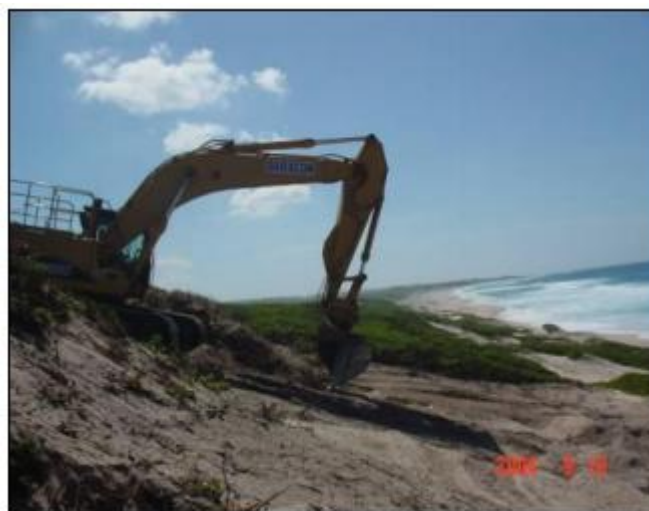
Figure 8. Excavator removing bitou bush.
