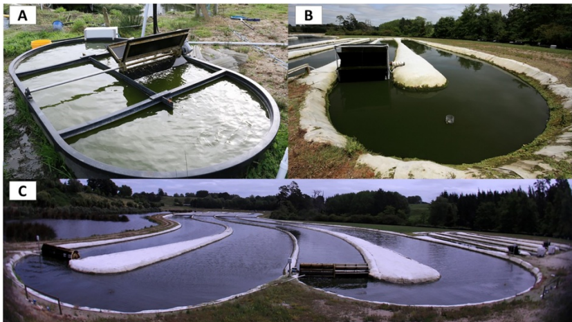
Figure 1. The different sized high rate algal ponds used in the experiment. A) Mesocosm pond with a total treatment volume of 1.5 m 3 , B) pilot-scale pond with a total treatment volume of 90 m 3 and C) two full-scale ponds with a total treatment volume of 2,900 m 3 each.
