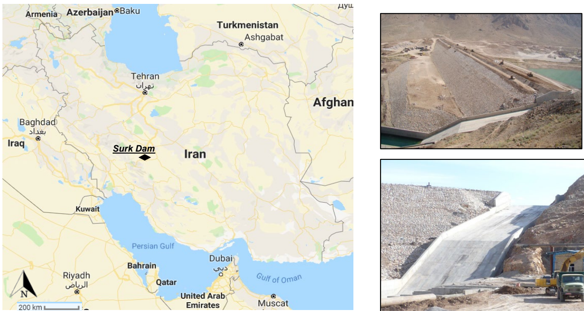
Fig 1. Location and view of Surk Dam body and spillway
