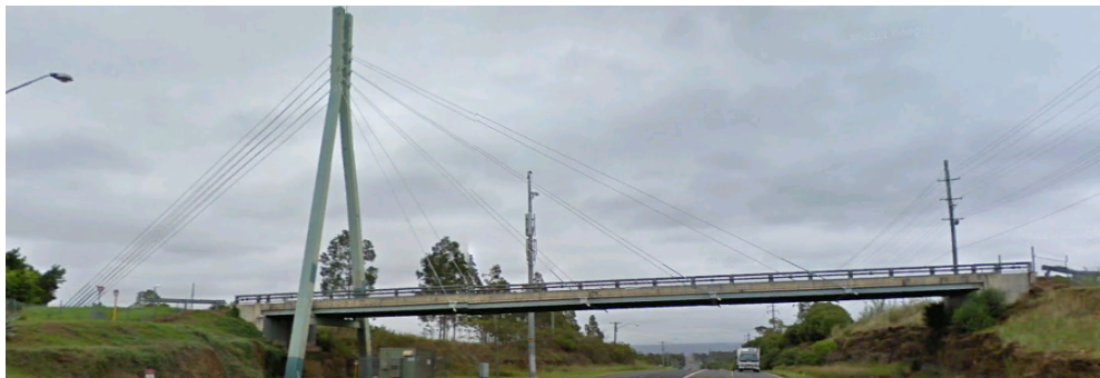
(a) The cable-stayed bridge
