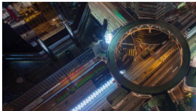
Figure 4. Pedestrian skyways in Hong Kong emerged from the stresses resulting from the growing population. 34
