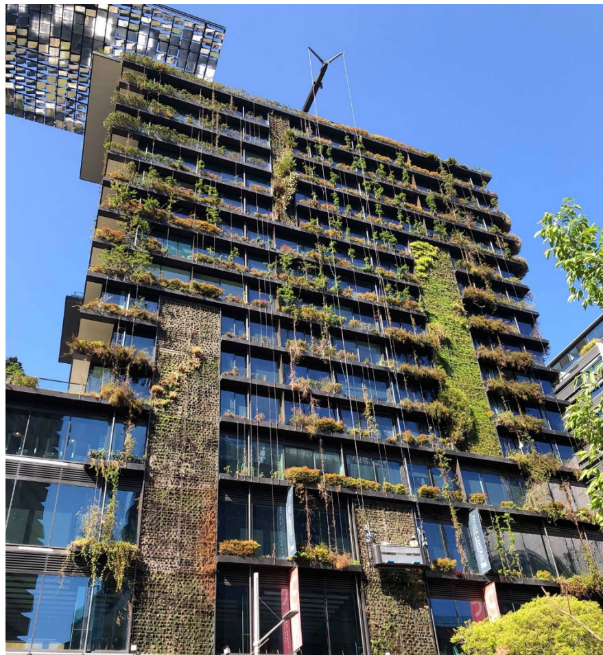
Plate 1 – existing methods of monitoring and maintaining green walls Central Park Sydney 2019
