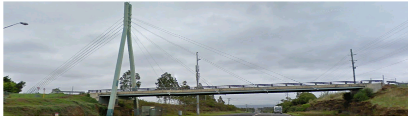
(a) The cable-stayed bridge
