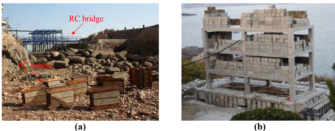
Figure 9: RC structures, RC beams and concrete prisms exposed on Xiaomai Island
