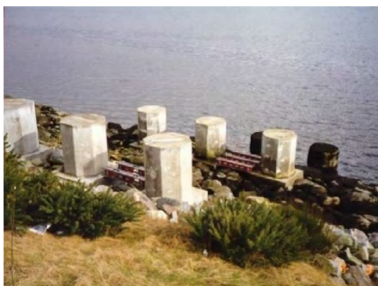
Figure 5: Concrete pier-stems exposed in Dornoch Firth [75]
