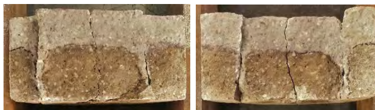
Figure 3: Chloride ingress into cross-sections 1 + 2 for CC-sample (lighter colour), D_{nssm} value affected by cracks
