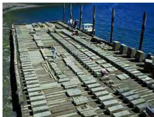
Figure 6: Concrete prisms and RC components exposed on Treat Island [87]
