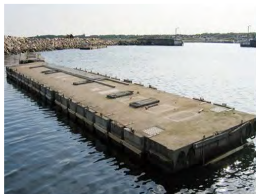
Figure 8: Concrete prisms and RC slabs exposed in Träslövsläge [66]
