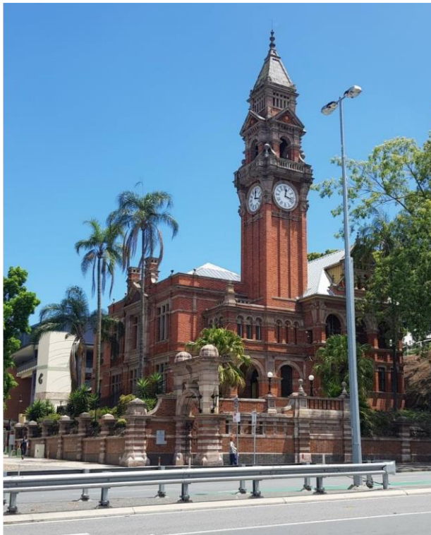
Fig. 4. South Brisbane Municipal Chambers
