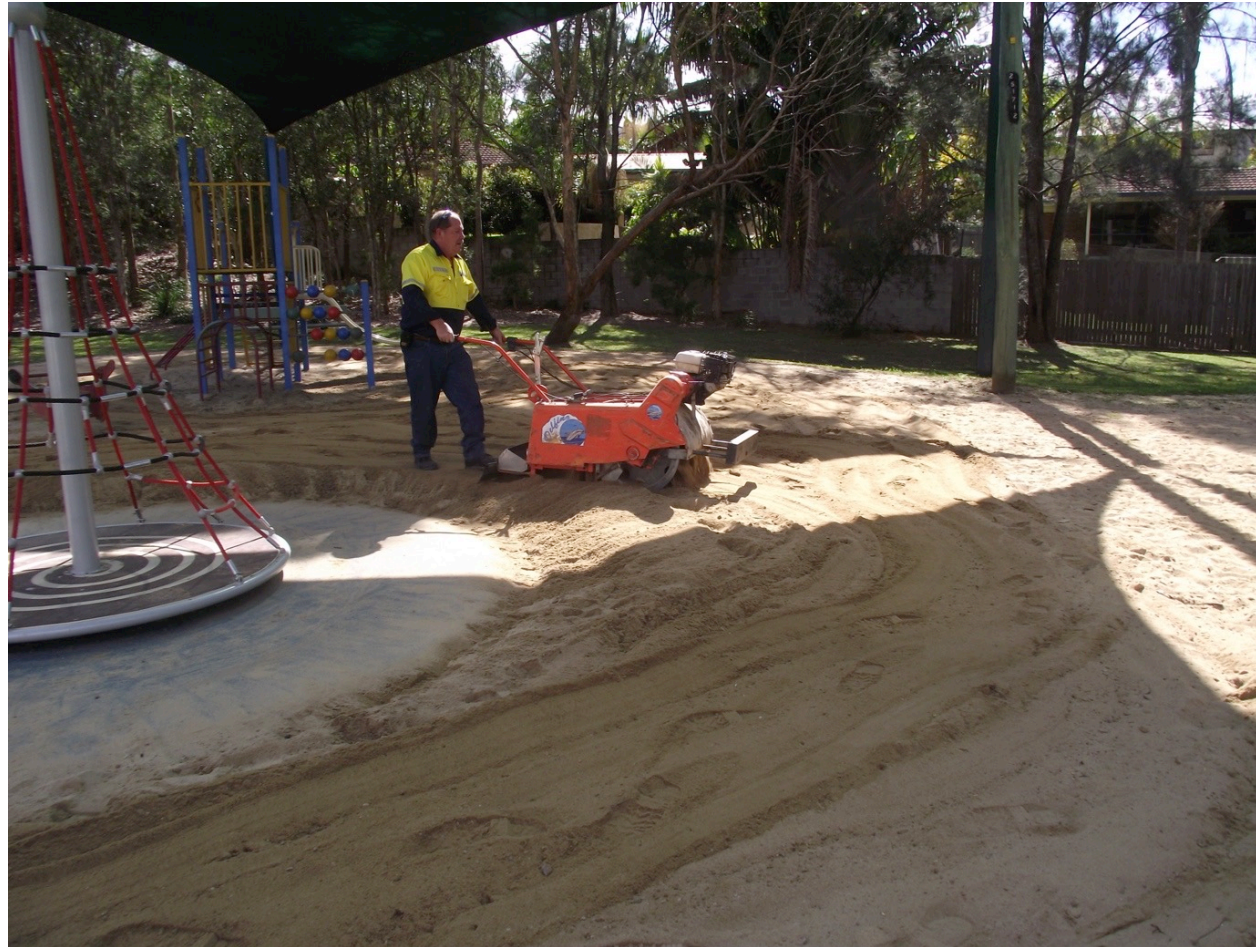
In-situ sieving using portable vibrating sieve
