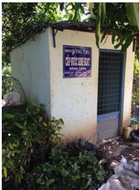
Figure 70 Song Thu pumping station
