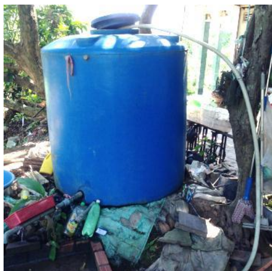
Figure 69. Example of a tank used by householders to store piped water to manage water pressure issues (Song Thu PE service area, Tan Phong Commune)
