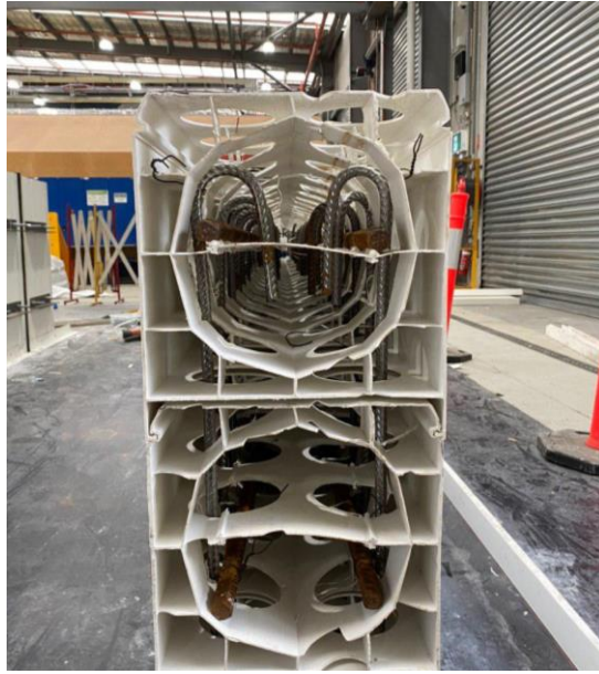
Figure 7: Dintel panels with shear and longitudinal steel reinforcements (before pouring concrete)
