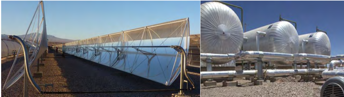
Figure 39: Trough collectors and thermal storage tanks at Minera El Tesoro. Reproduced from Abengoa.
