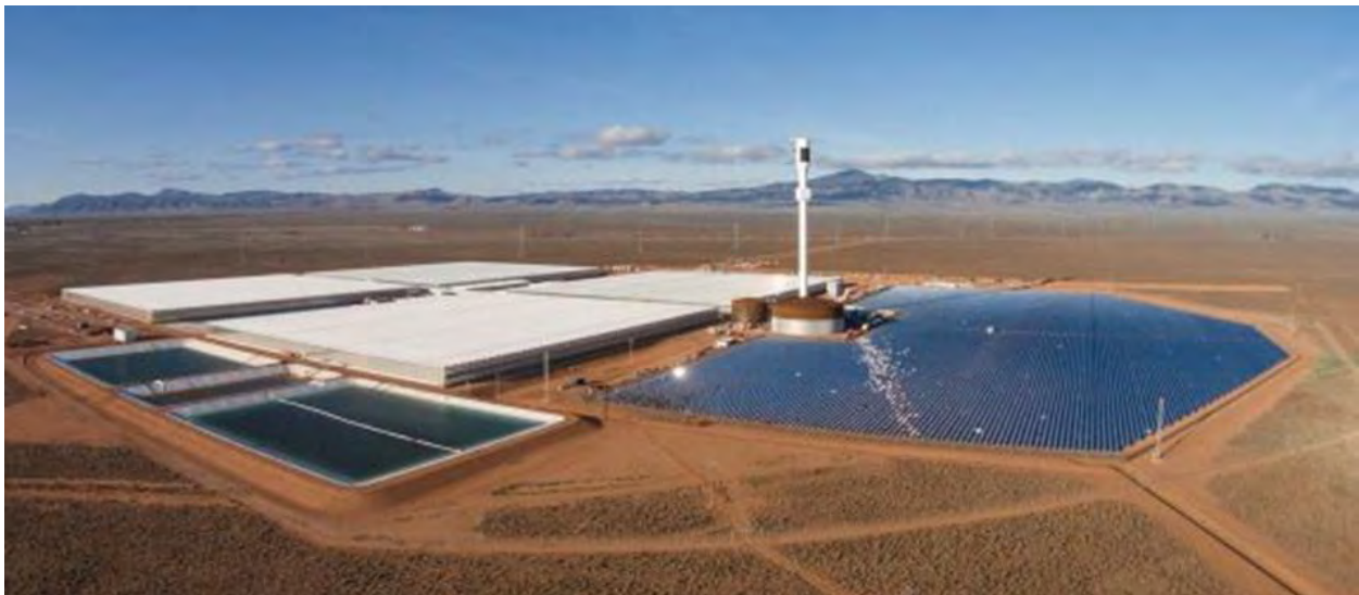
Figure 18: Sundrop Farms greenhouses and concentrating solar power plant (image Aalborg CSP).
