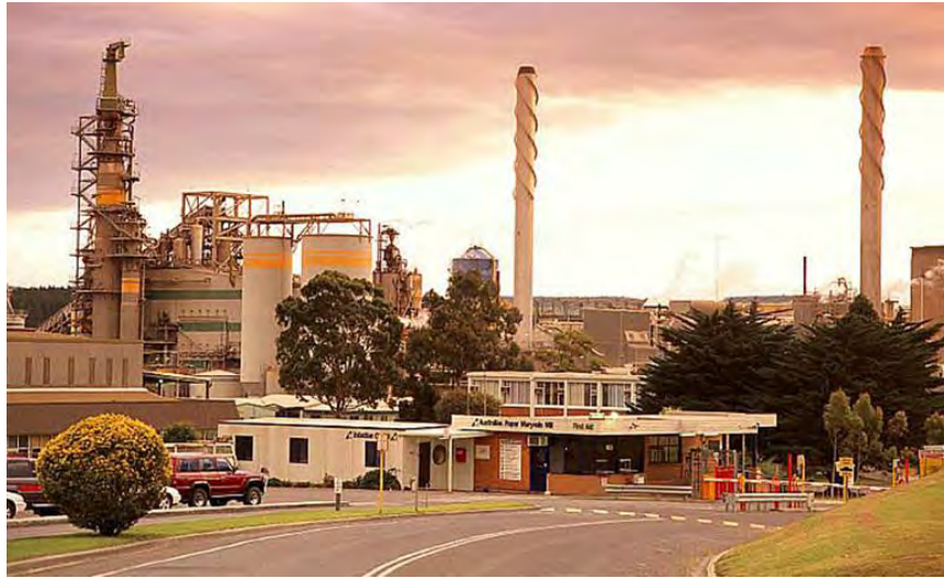
Figure 64: Australian Paper's Maryvale plant. (image from sprinter.com.au .)
