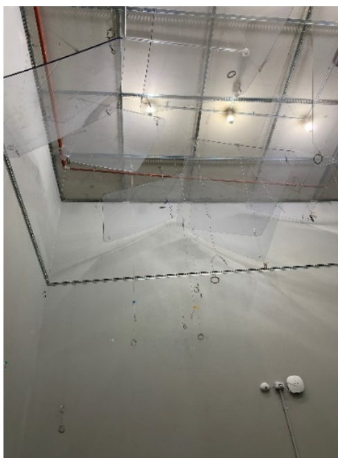
Figure 2: Six diffusers with relatively lower heights to the floor were removed for the measurement with 14 diffusers.
