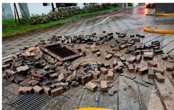
**Figure 2.** Pothole due to lightning strikes in Batok Town, Bukit, Singapore.
