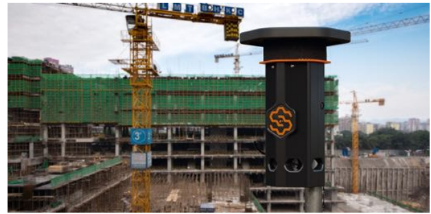
Figure 17. SiteHive Hexanode in normal operating position when deployed on a construction site.
