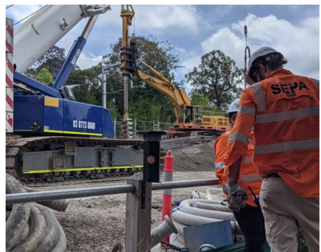
Figure 2. SiteHive Hexanode testing on a construction site.
