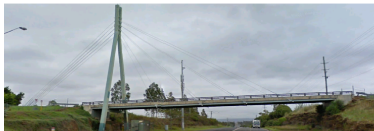
(a) The cable-stayed bridge
