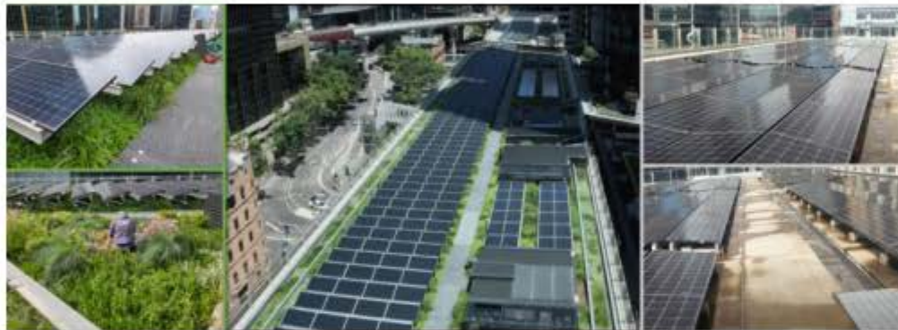
Figure 1: Aerial imagery of study site. Daramu house (green roof) featured in the foreground and International house (conventional roof) featured in the background. The sister buildings are near-identical with differences (excluding greenery) owing to building maintenance unit design, rooftop infrastructure, and solar panel layout.
