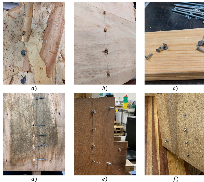
Figure 14. Photos of STC failures on (a) OS8, (b) & (c) HP6, (d) WSP5, (e) WWU7, and (f) WPB5.
