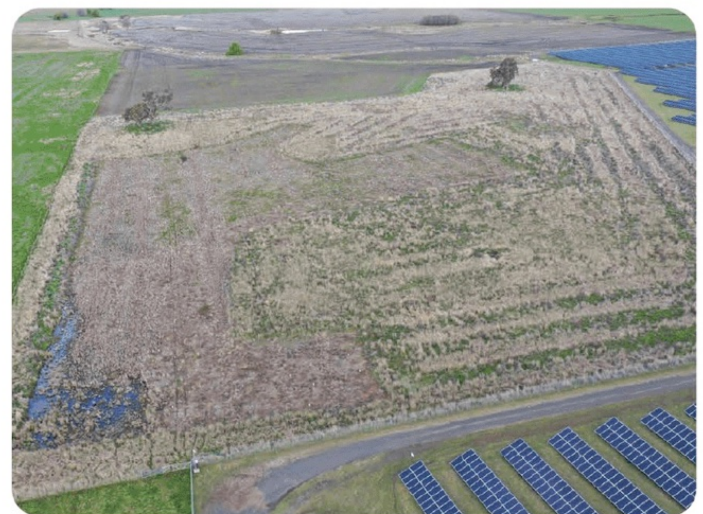
Areas adjacent to the solar arrays on White Rock Solar Farm (west of Glen Innes) have been set aside for revegetation as part of the project's biodiversity offsets.
