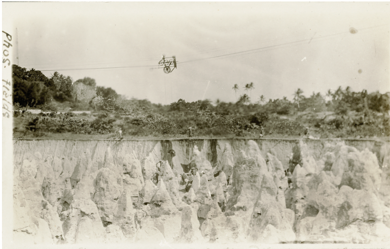
Figure 8. The overhead cableway at Banaba in c.1913 designed by the Australian engineering firm J. M. and H. E. Coane. Phosphate deposits can be seen in the background, behind the coral pinnacles left behind following extraction. Source: Phosphate Fields, Banaba, Kiribati, PIC Album 1203, National Library of Australia.
