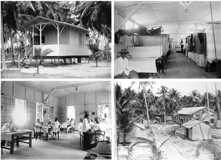
Figure 6. Photographs of prefabricated buildings on Nauru manufactured by F. H. Schmidt in Altona-Hamburg. Depicted are an officer's dwelling (top left), the interior of one of the island's numerous "Coolie Barracks" (top right), the island hospital (bottom right) and the interior of the mess hall for exclusive use by white employees of the PPC (bottom left). Source: Nauru Photos Attached to Report by A. H. Gaze, 1907, NAA 671741.
