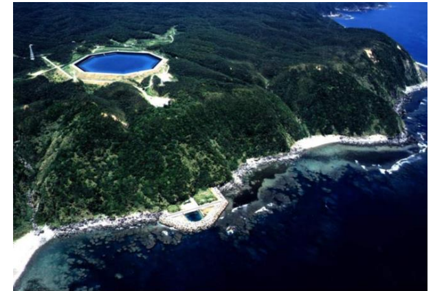
Yanbaru seawater PHS plant on Okinawa Island, Japan
