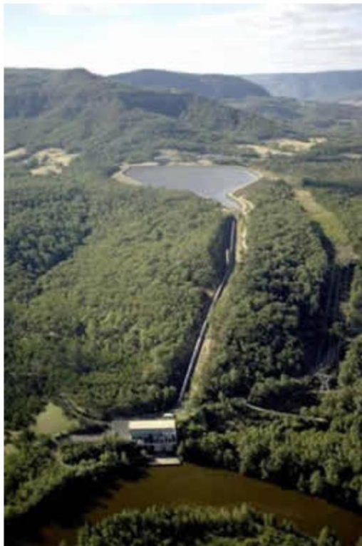
Shoalhaven Scheme – Bendeela Pondage, Australia
