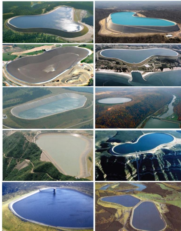
Turkey nest type PHS systems – Goldisthal, Avce, Dlouhé Stráně, Tianhuangping, Turlough Hill, Coo-Trois-Ponts, La Muela, Seneca, Ludington, Taum Sauk.
