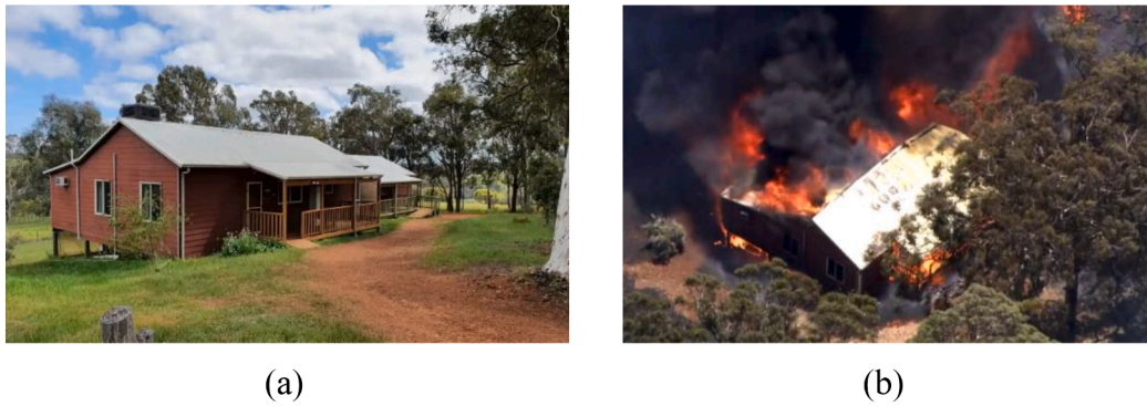
Fig. 4. (a) The house before the fire [51]; (b) in the fire [50].
