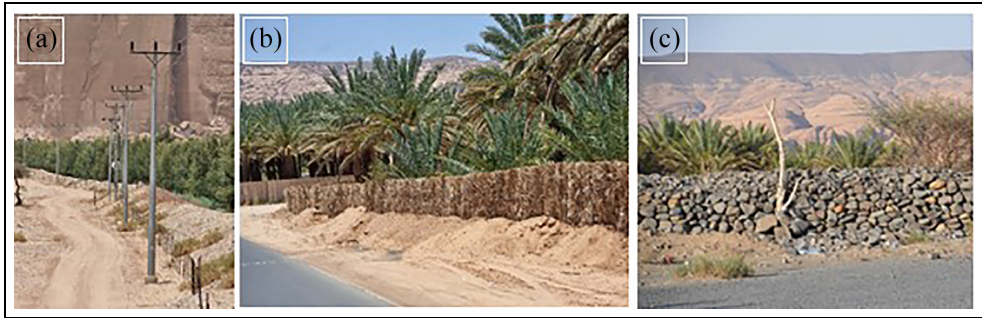
Figure 2. The traditional techniques for mitigating flash floods, erosion and desertification. (a) Oqoom ; (b) a combination of oqoom and washea . (c) A traditional stone wall (by the author).
