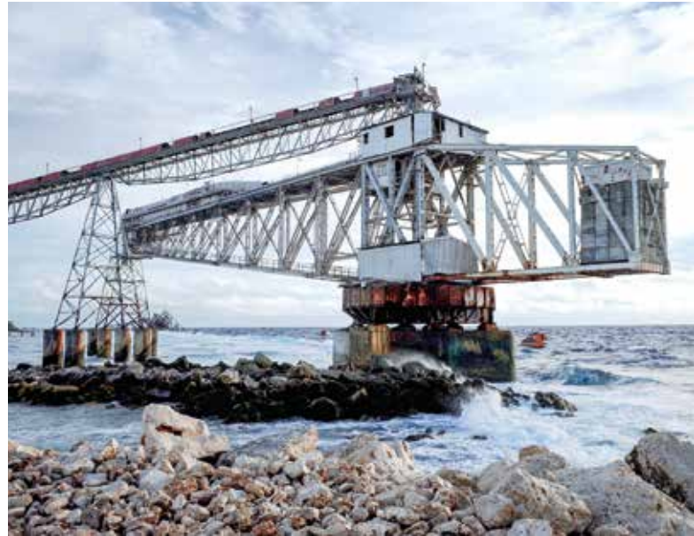
Fig. 15 One of two pivoting steel cantilevers currently used by the Republic of Nauru Phosphate Corporation to load ships in the deeper water off the coral reef, 2023
