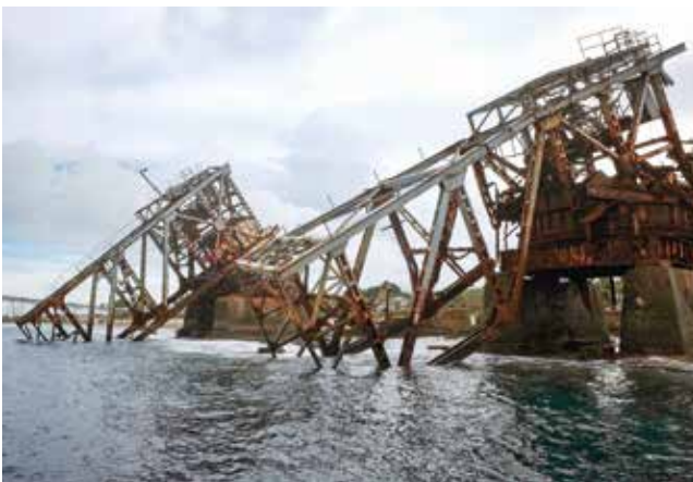
Fig. 8 Steel cantilevers sit collapsed on the coral reef, 2023
