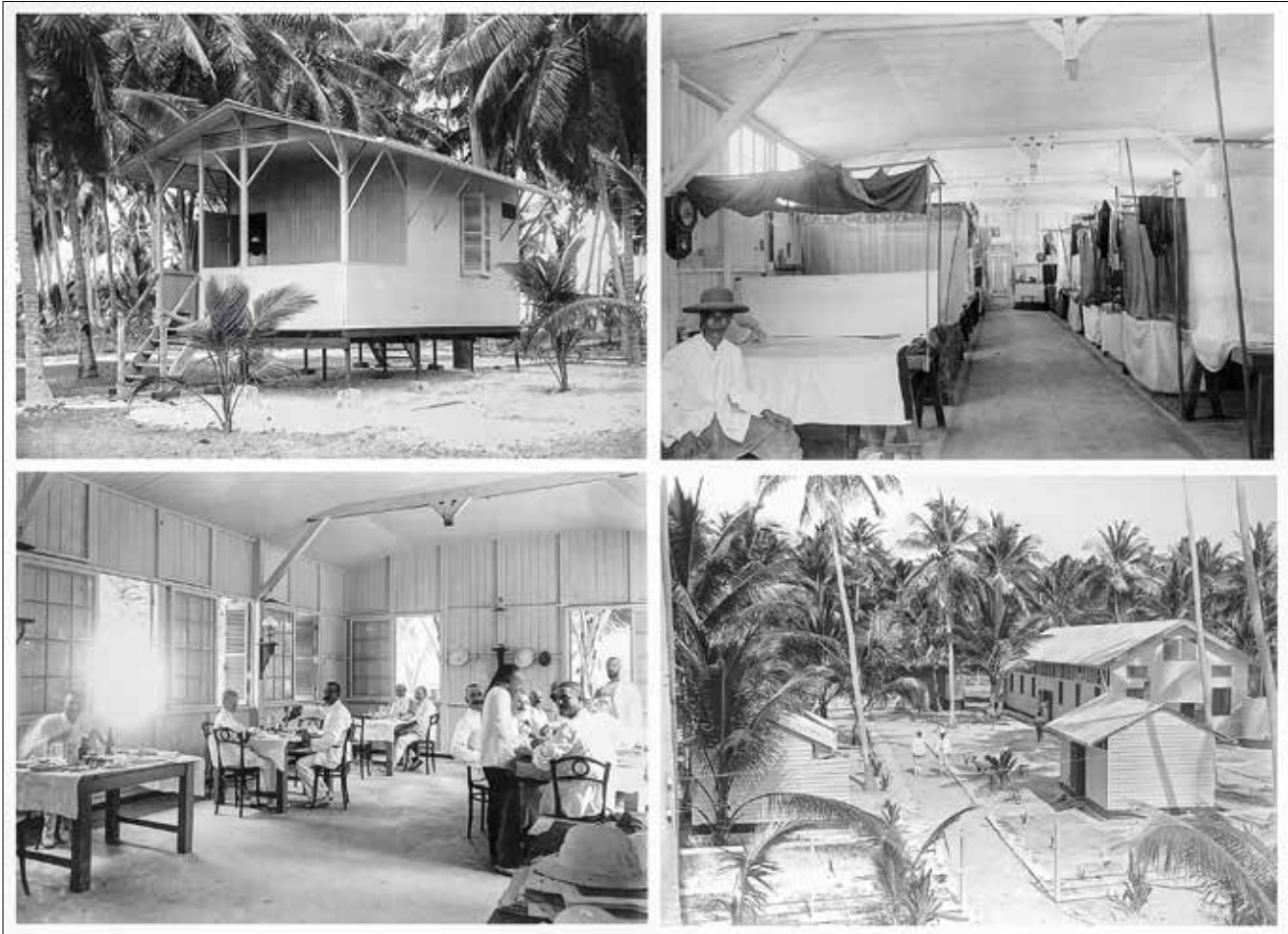
Fig. 7 Prefabricated buildings on Nauru manufactured by F. H. Schmidt of Hamburg-Altona. Depicted are an officer's dwelling (top left), the "Coolie Barracks" (top right), the island hospital (bottom right) and the mess hall (bottom left), 1907
