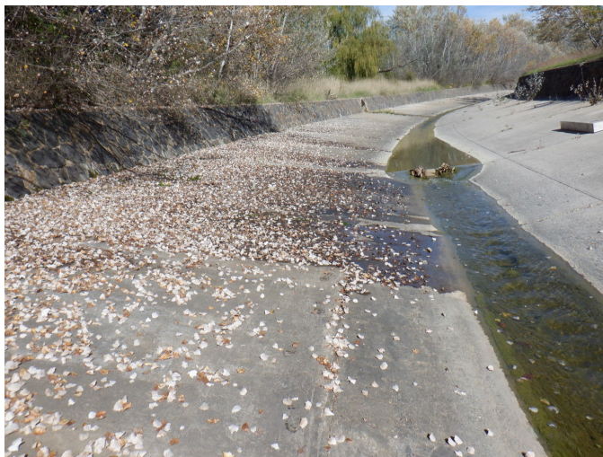
Figure 8. From Subsurface water flowing through concrete into Yarralumla Creek [Photograph], K. Harriden, n.d. Used with permission of the photographer.
