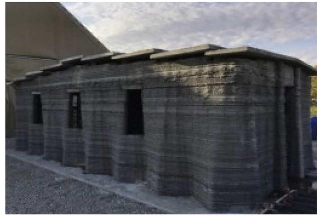
(b) B-Hut structures with Chevron wall geometry [102]
