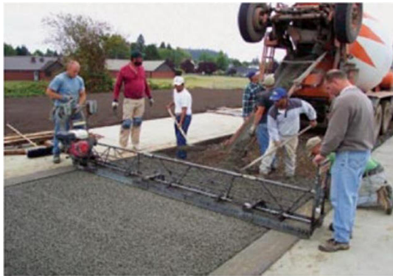
Figure 2.25 Placing pervious concrete [2]
