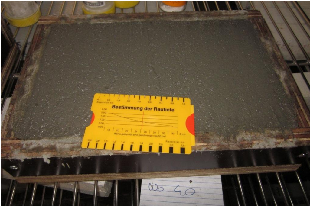
Figure A. 10. Early age cracking of Wo4.0 sample after 24 hours
