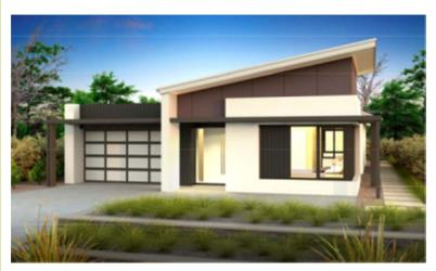
The Eco-living Net Zero Emissions Home is a collaboration between Clarendon Homes (the builder) and Landcom (the land and funding provider). The home has a modelled 8-star NatHERS rating and is aimed to appeal to the project home market. Inclusion of a solar electricity generation system and energy efficient appliances complete the homes net zero carbon occupied design. The main features include:
