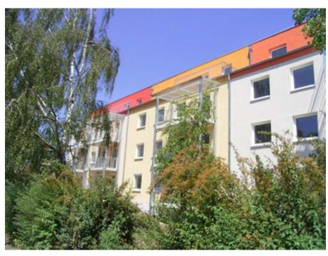
This renovation of two postwar apartment buildings in Frankfurt achieved a 94% reduction in heating demand and almost met the Passivhaus Standard, which is impressive for a renovation in an apartment building. The buildings contained 60 apartments and were in a bad state. The renovated buildings contain 53 apartments ranging from 33 to 100 m<sup>2</sup> in size. Key features of the renovation included:
