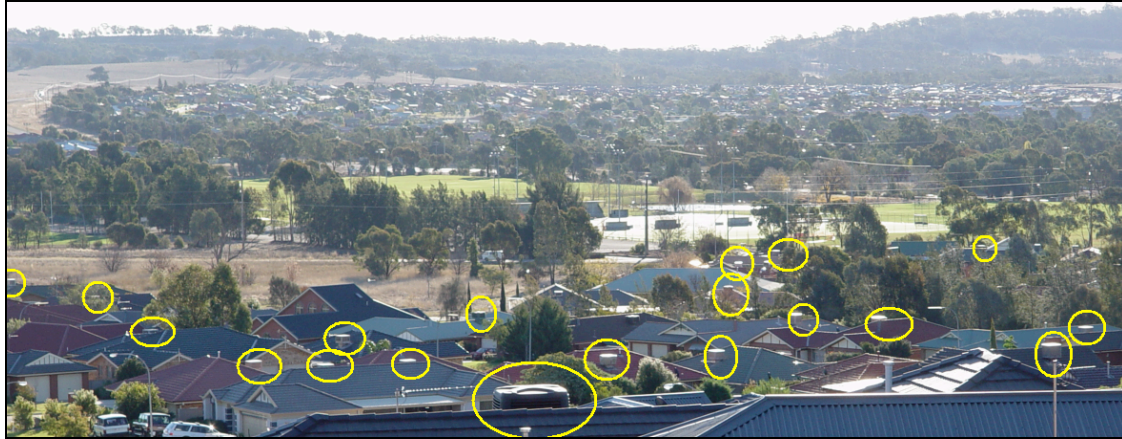
Figure 7: Photograph of EACs installed on new homes in Wagga Wagga (EACs are circled in yellow). Source: provided by Greg Finlayson, Riverina Water.
