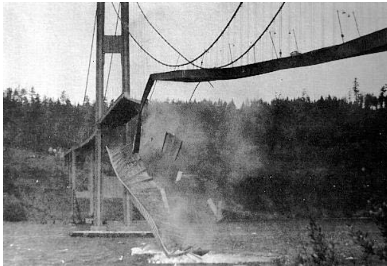
Figure 1-4 Zipper-type collapse of the Tacoma Narrows Bridge (Starossek, 2011).
