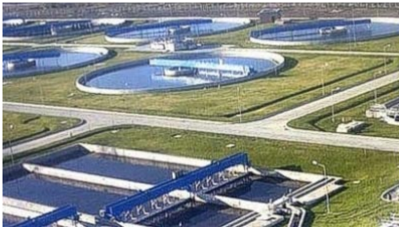
Figure 4-2 Activated sludge system aerial view (SPG Media Limited. 2006a)
