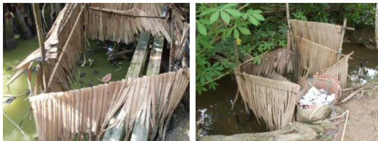
Figure 18 Typical shared hanging fishpond toilets in the Mekong
