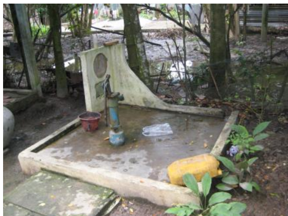
Figure 15 Functioning bore well
