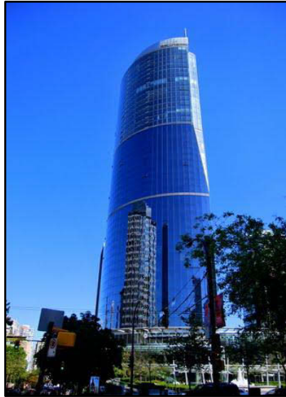
Figure 2.7. One Wall Centre in Vancouver, equipped with tuned liquid dampers at the top storey
