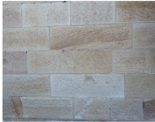
Figure 2.2 Plain ashlar masonry
