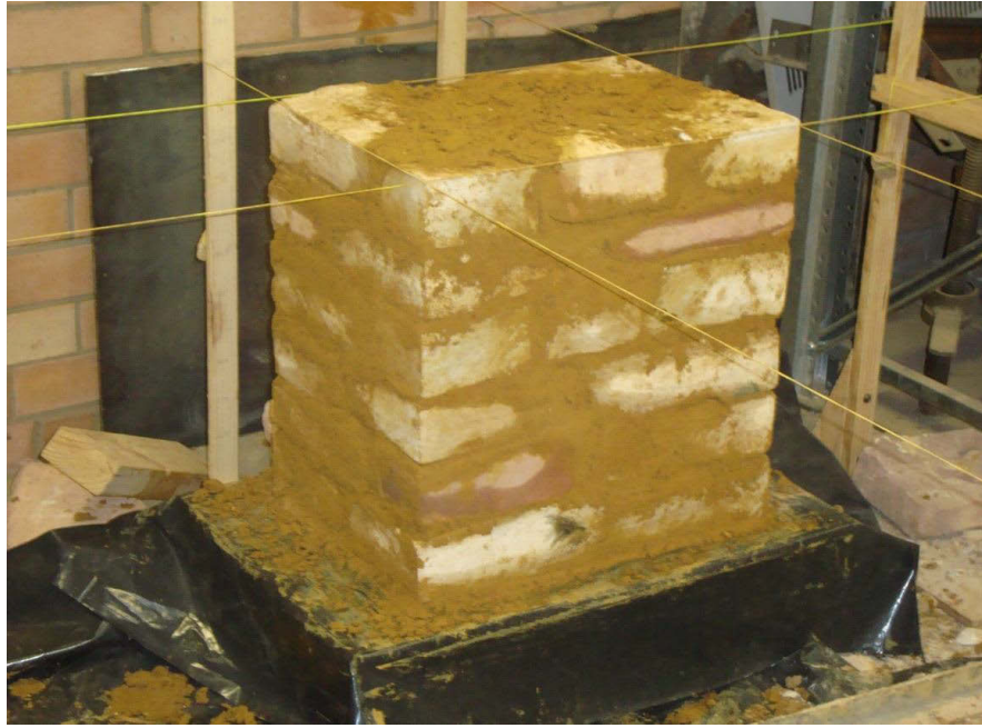
Figure 5.3 Wall specimen during construction
