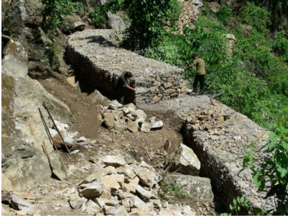
Figure 3.5 Gabion wall during construction ( Photo: U. Dackermann )
