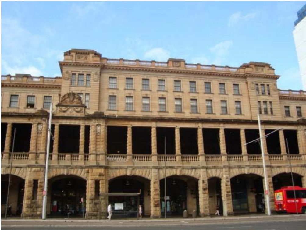
Figure 1.1 Stone masonry building in Sydney
