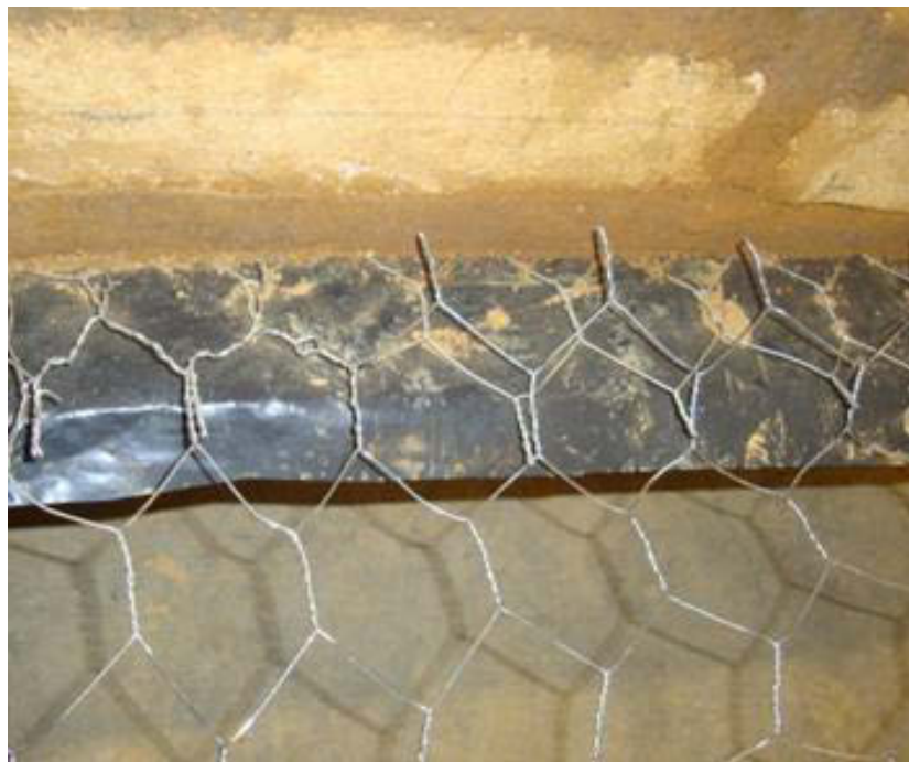
(d) Completed up to fourth side from left end
