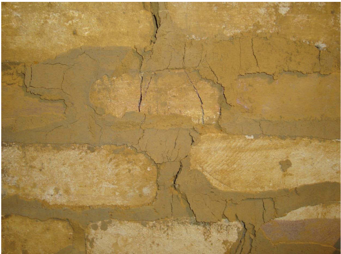
Figure 7.8 Close up view of mortar joint in rubble masonry
