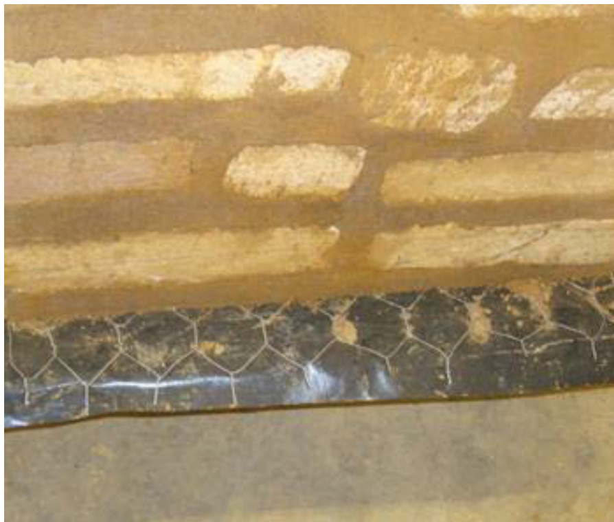
Figure 5.9 Alignment of bottom mesh
