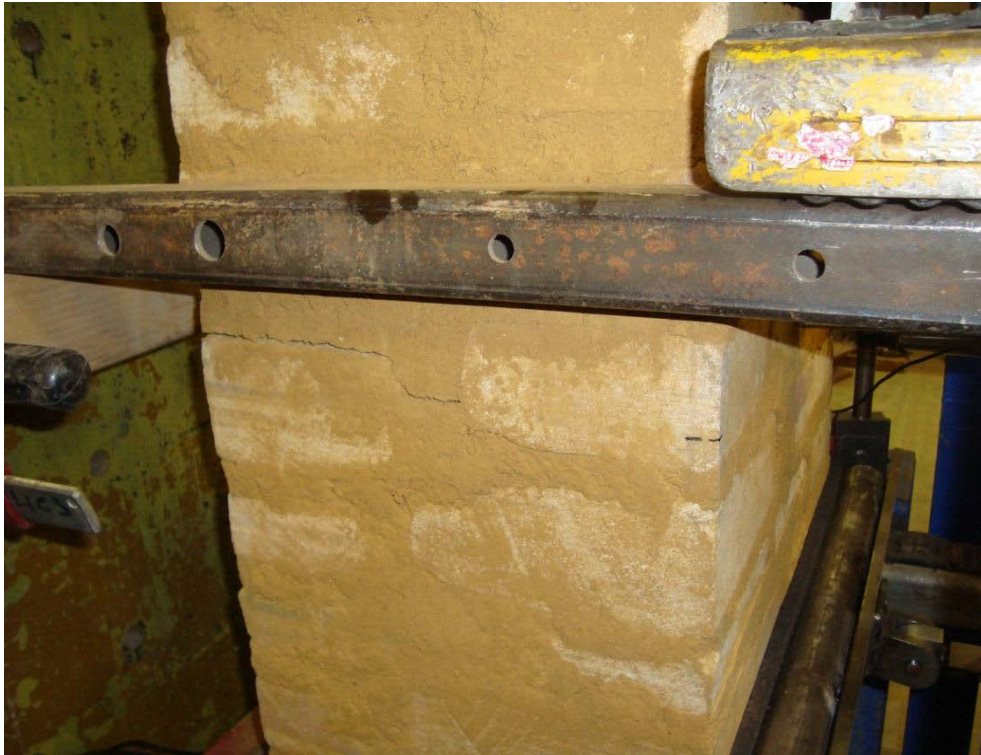
Figure 5.37 Crack in unreinforced wall specimen (Bending in vertical span)
