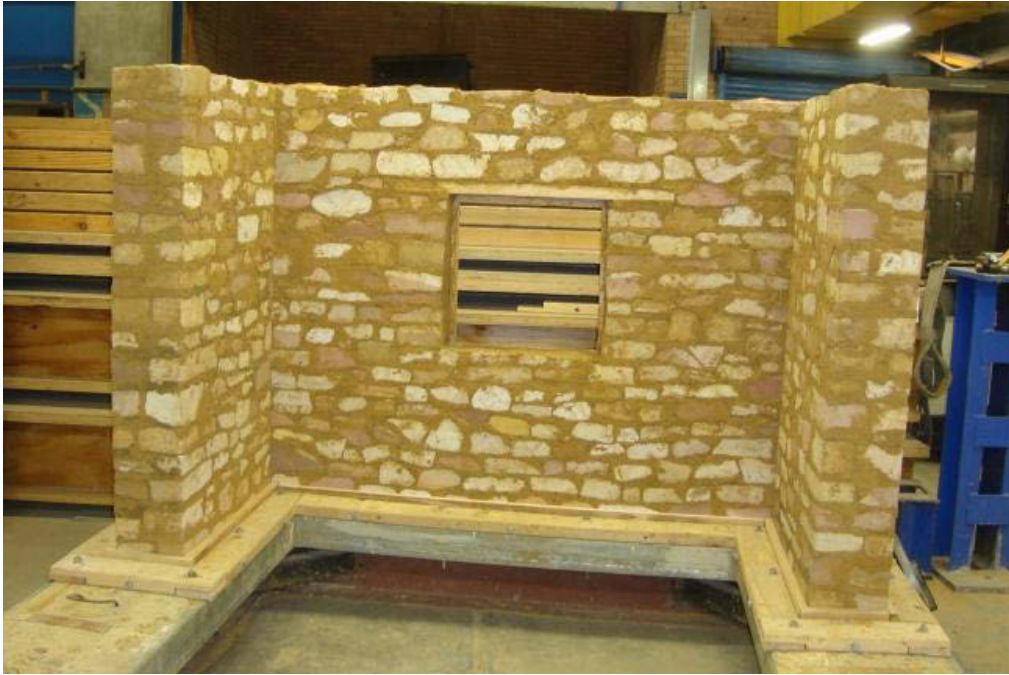
Figure 5.23 Clamping system at the bottom of the specimen
