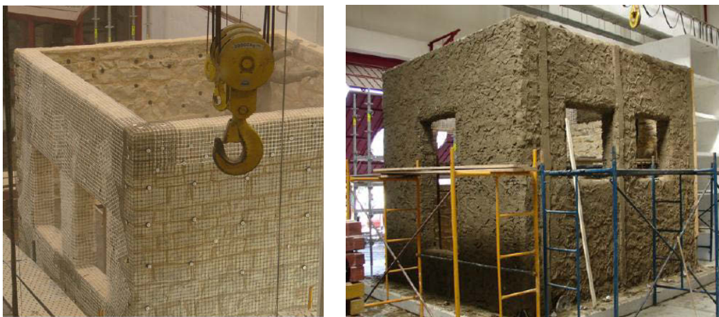
(a) after placing vertical reinforcement (b) covered with mortar
