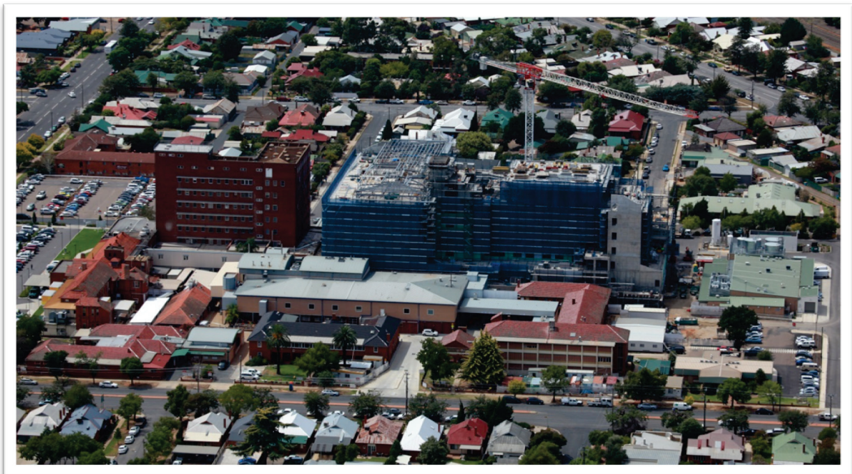
Figure 6: Wagga Wagga Base Hospital. Photo supplied by City of Wagga Wagga.
