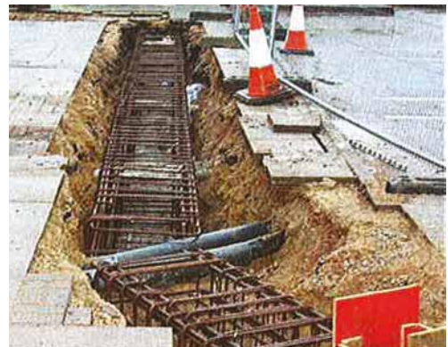
VSB foundations around underground services
