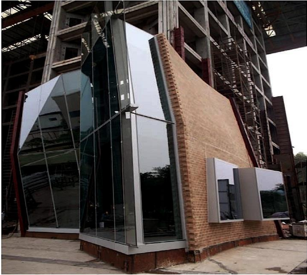
Figure 2. Finished mock-up prior to testing.
