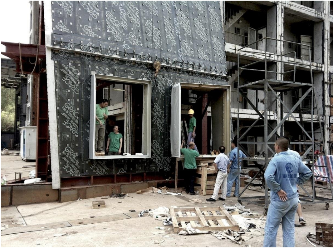
Figure 1. Performance mock-up under construction in China.
