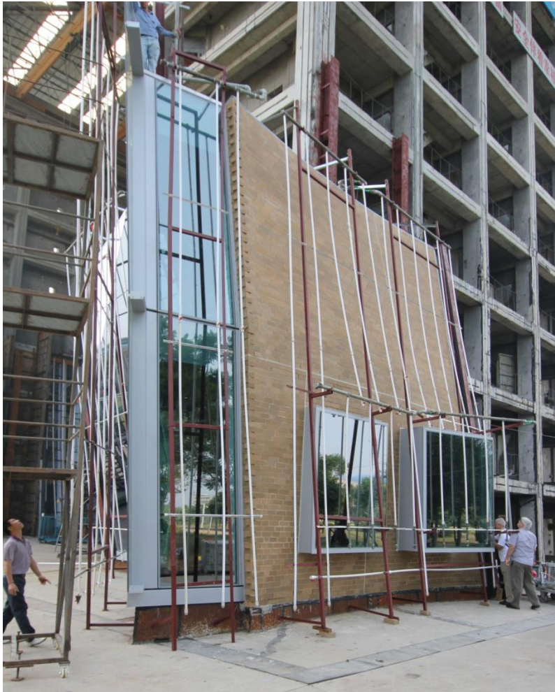
Figure 3. Testing rigs to direct water and air onto the façade being put into position.
