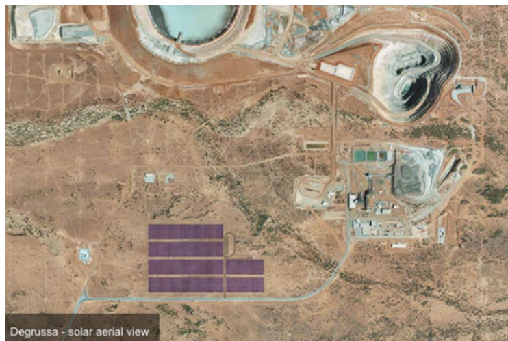
Figure 21: Aerial view of the DeGrussa Mine near Meekatharra
