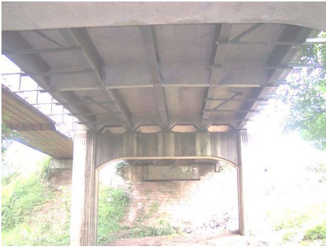
Figure 6. Underside of Redbank Creek bridge
